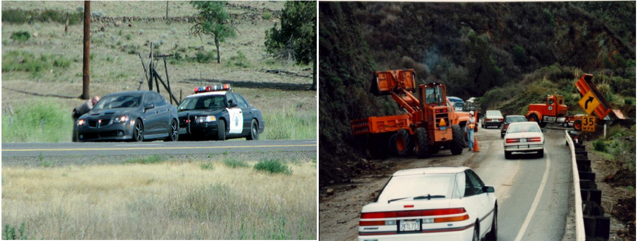
Figure 9 Shoulders allow for law enforcement and maintenance activities
