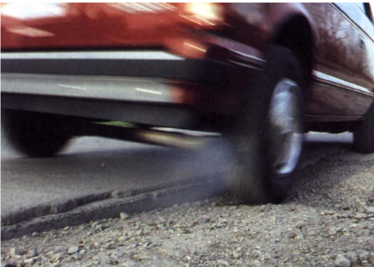
Figure 18: Shoulder drop-offs can lead to crashes
