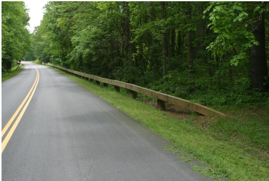
Figure 19: Roadside barrier shielding trees
