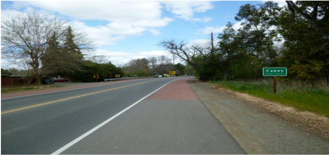
Figure 17: Paved shoulders with contrasting color
