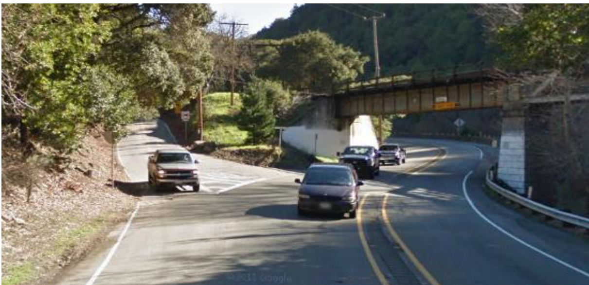
Figure 15: Palomares Rd. Intersection and Farwell Undercrossing
